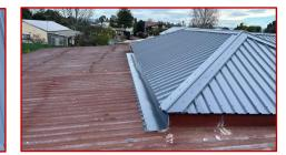
Things are beginning to wrap up and come to a close. The work on all the roofs that we are doing now, is done apart from a piece of flashing that needs to be completed after the guttering is done. Extra flashings were laid around where the metal was badly rusted near the skylights – a roof that we are not getting replaced at this
